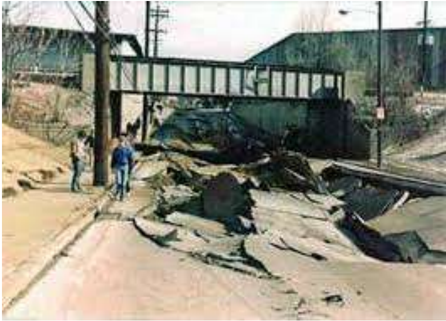
Illegal hexane release into the sewer from Ralston Purina soybean plant in Louisville Kentucky 1981
