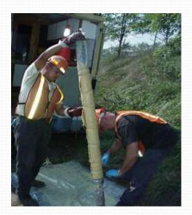
• Short liner spot repairs to rehabilitate holes, cracks and eliminate sources of heavy infiltration.
