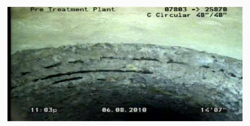
H<sub>2</sub>S GAS IS PRODUCED BY THE SLIME LAYER UNDER THE WATER LINE. IT IS THEN OXIDIZED TO SULFURIC ACID BY THIOBACILLUS BACTERIA LIVING ON THE NON-SUBMERGED SURFACES, WHICH THEN 'EATS' THE CONCRETE, EXPOSING THE REBAR REINFORCEMENT, AND CAN LEAD TO COLLAPSE OF THE PIPE.
