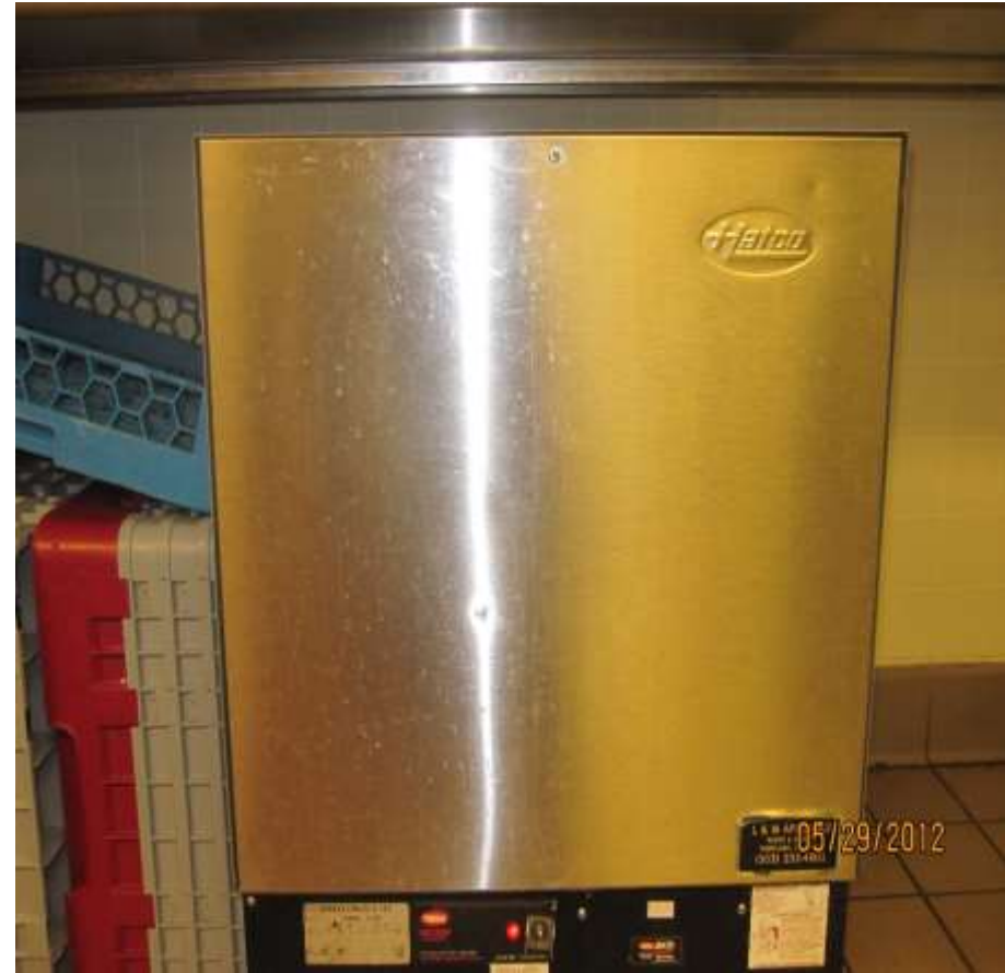
Water Heater Booster
