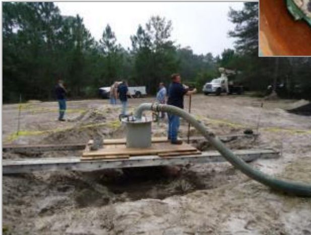
Downstream Access Tap & Flow Diversion
